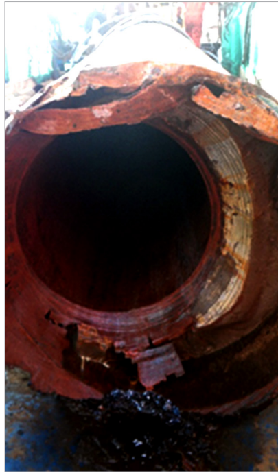
Successfully cut through cemented 13 3 / 8 -in. and 20-in. casing strings downhole.
