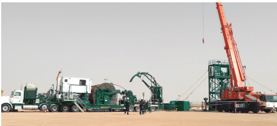
The TransCoil rigless-deployed ESP system is installed in a well in the Middle East.
