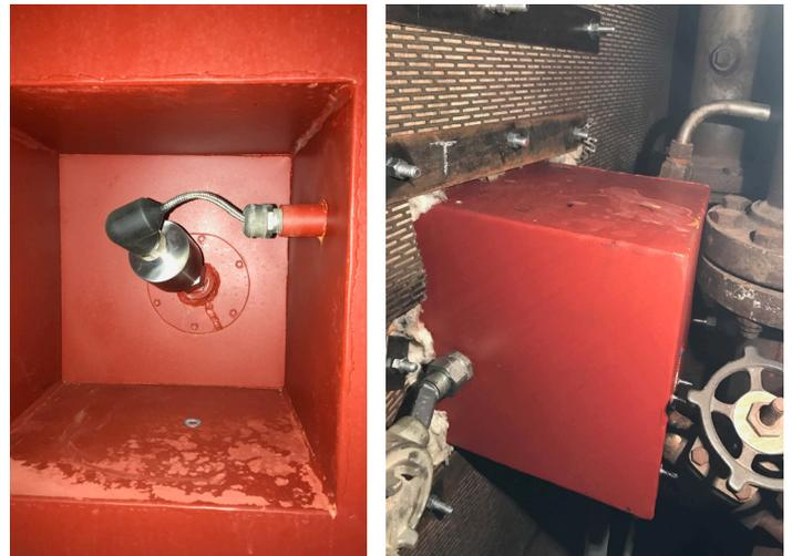
*This new cost-effective installation offers the lower cost Flame Tracker option with no water-cooling system needed. Flame Trackers are exceptionally reliable and can be a big improvement over older Geiger Muller-type sensors or other less effective sensing methods. Reuter-Stokes is pleased to share drawings and installation methods with new customers, including the installation of Flame Trackers on turbines with no recessed panels or turbines that include panels.*
